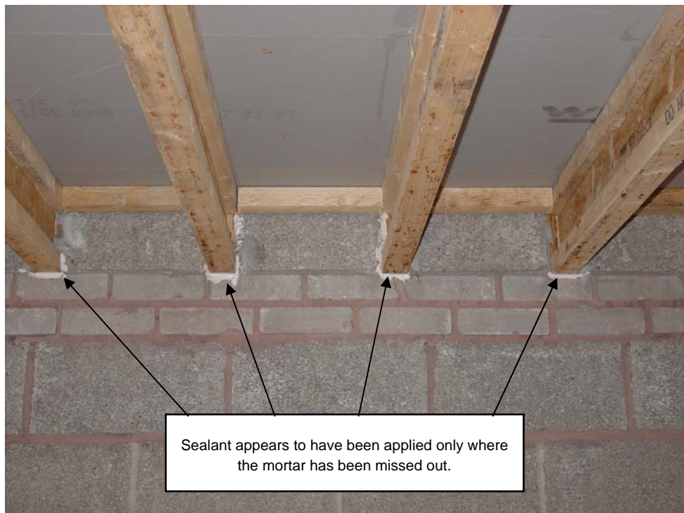
Figure 1 Partial application of mastic sealant (developer B).
