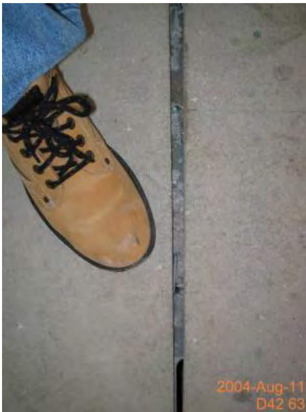
Figure 18 Leaks at the junction between flooring panels.
