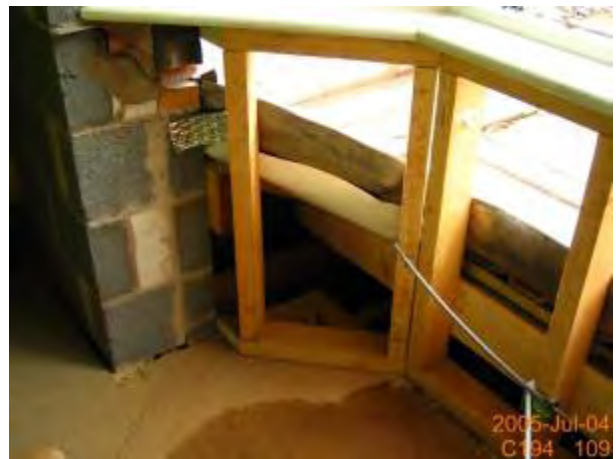
Figure 11 Developer C's detached property, C194, and internal view of partially constructed first floor bay.
