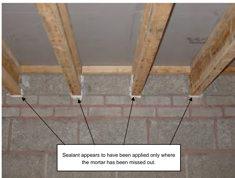
Figure 1 Partial application of mastic sealant (developer B).
