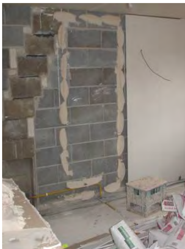
Figure 9 Discontinuous ribbons of adhesive used to seal plasterboard dry-lining.
