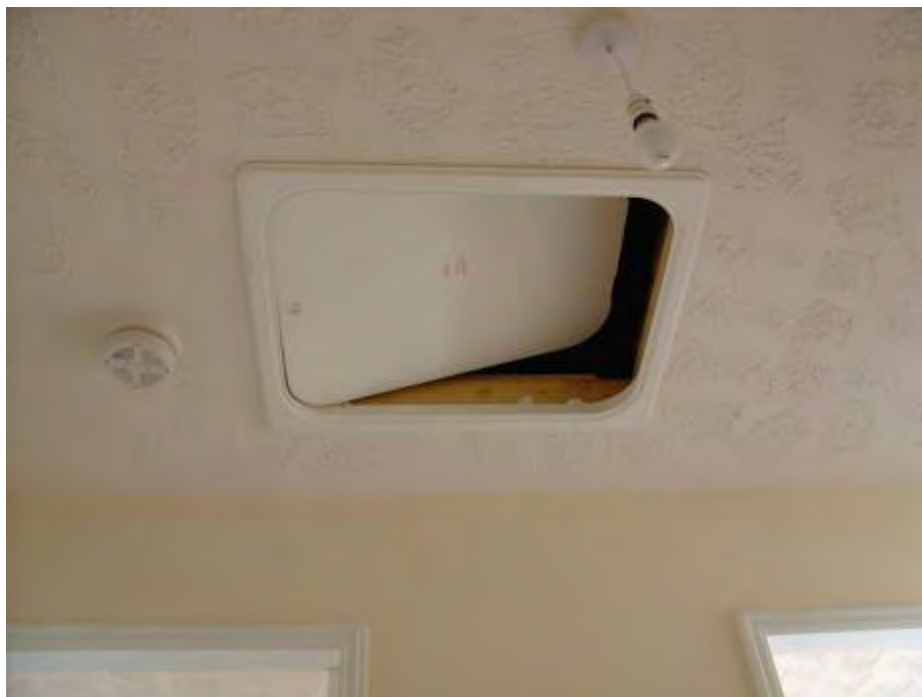
Figure 32 Loft hatch lifting during pressurisation test.
