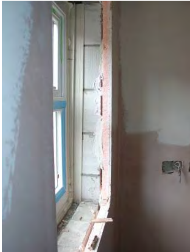
Figure 10 Discontinuous ribbons of adhesive around window opening.
