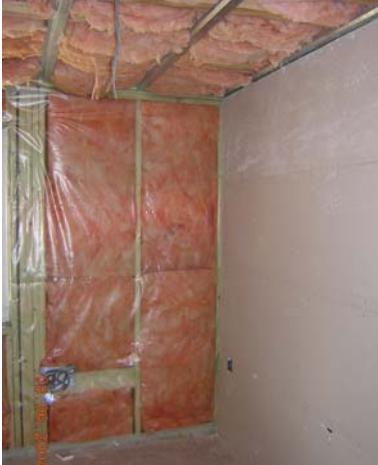
Figure 3.75 High timber concentration at window jamb.
