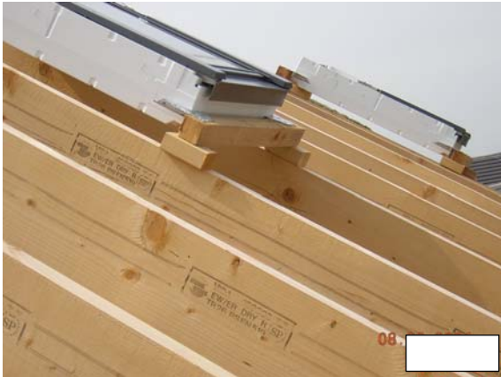
Figure 3.60 Rooflight fixed above external insulation to rafters.
