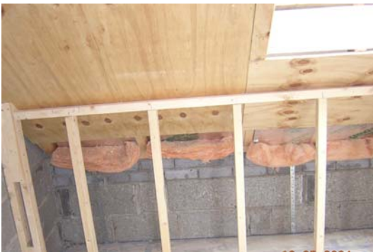
Figure 3.58 Cavity wall – roof junction.
