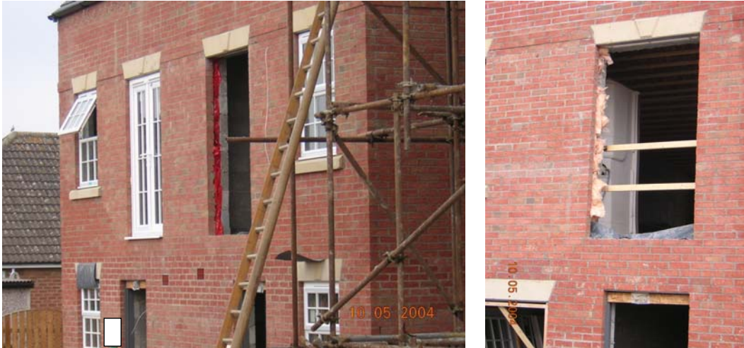
Figures 3.37 and 3.38 Alternatives to proprietary cavity closers.
