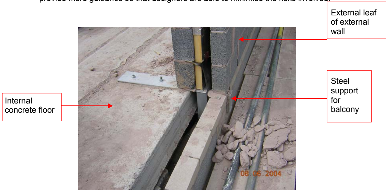
Figure 3.33 Balcony support through partial-fill masonry construction.
