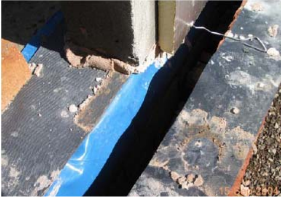
Figures 3.08 and 3.09 Partial-fill masonry construction, slab edge detail.
