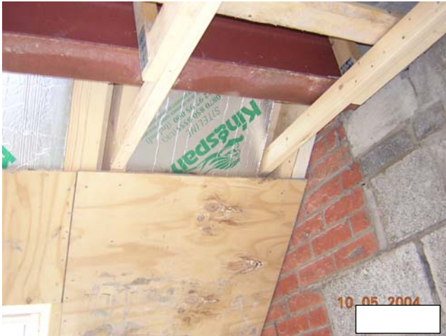
Figure 3.51 Ventilated rafter void all insulation between rafters.
