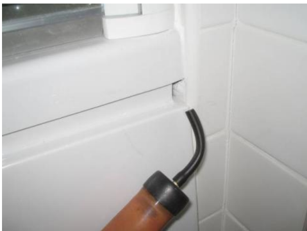
Figure 20 – Leakage at Bath Surround and Sink Boxing-in
