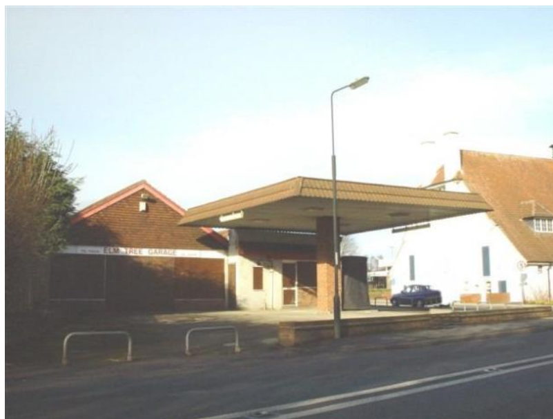
Figure 2 – Elm Tree Garage in New Earswick Prior to Demolition
