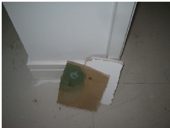
Figure 106 – Plasterboard Stained by Leak from Solar Pipe
