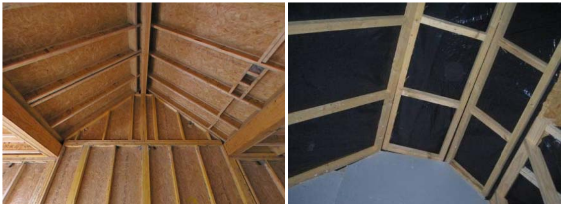
Figure 55 – Construction of Ceiling and Roof Void
