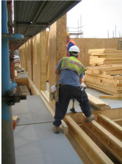
Figure 52 – Installation of First Floor Timber Frame Panels
