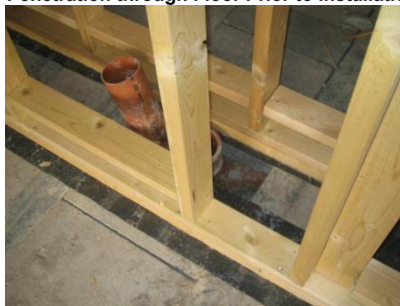
Figure 49 – Soil Pipe Penetrations through Ground Floor Prior to being Boxed-in
