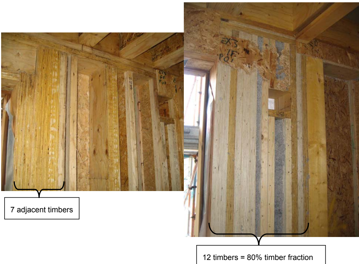
Figure 60 – Exposed External Timber Panels Showing Additional Timber
