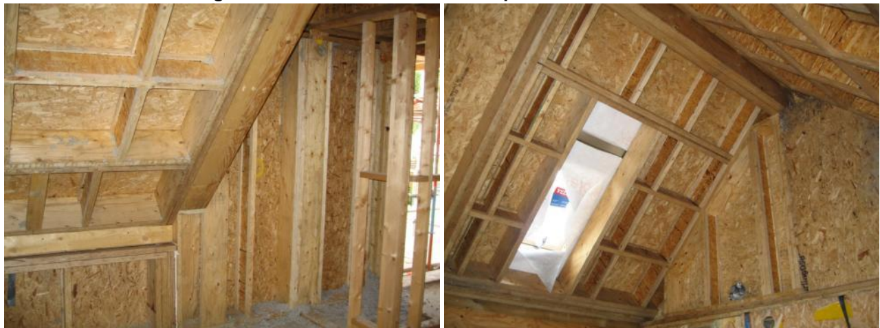
Figure 65 – Additional Timber in Exposed Roof Panels
