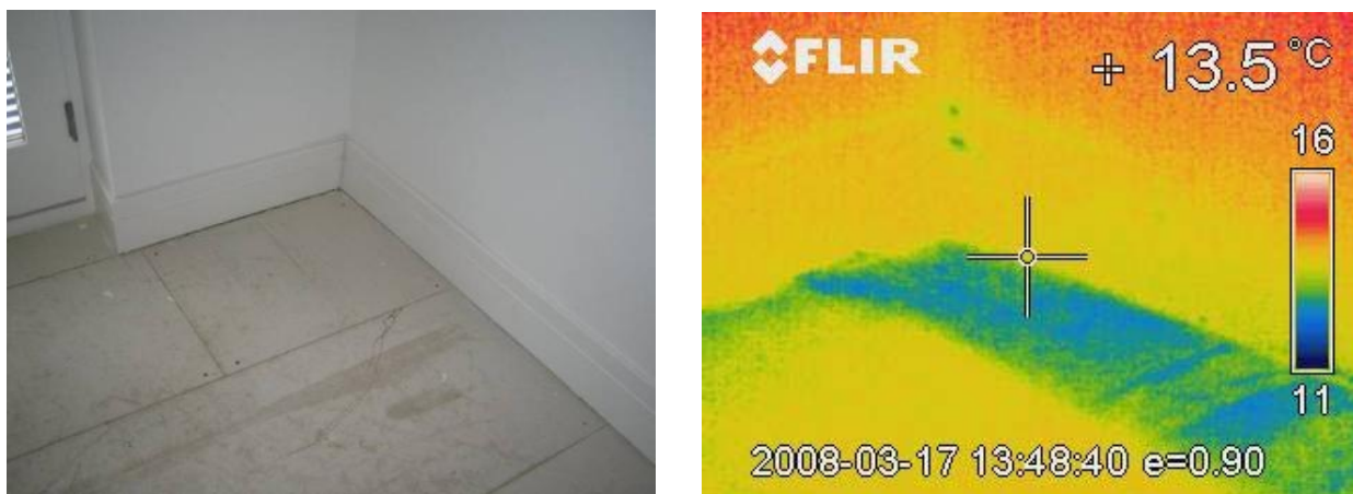
Figure 40 – Floor of Bedroom on First Floor of House F
