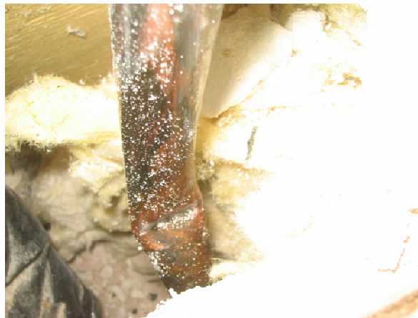
Figure 106 – Plasterboard Stained by Leak from Solar Pipe
