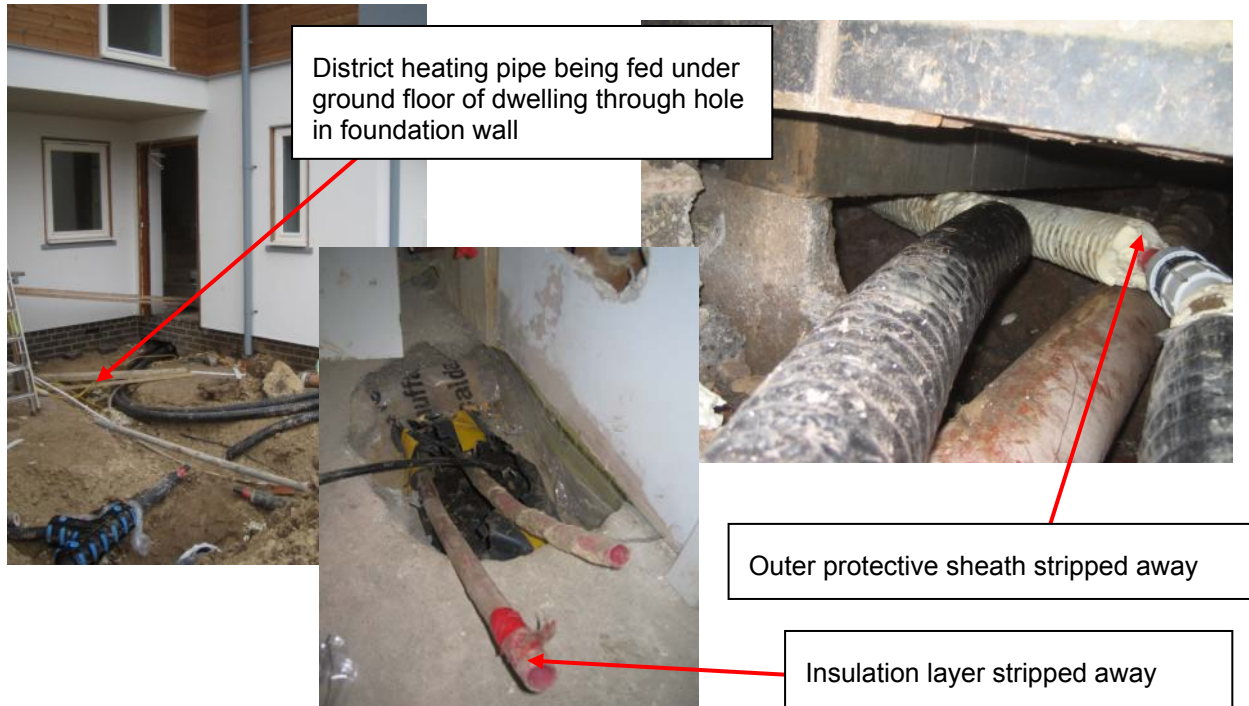
Figure 70 – Installation of District Heating Pipework
