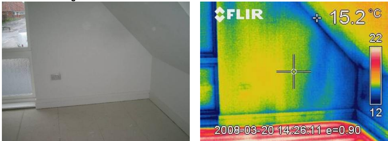
Figure 44 – Gable Wall of House D in Bedroom above Plant Room
