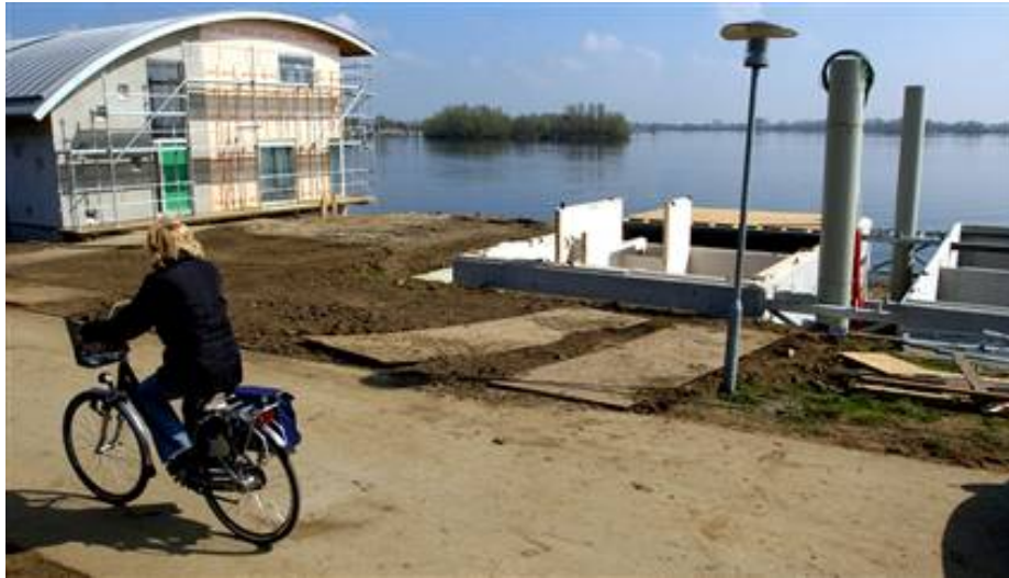
Figure 10 - Floating Homes Being Constructed in the Netherlands (Deutsch 2004)
