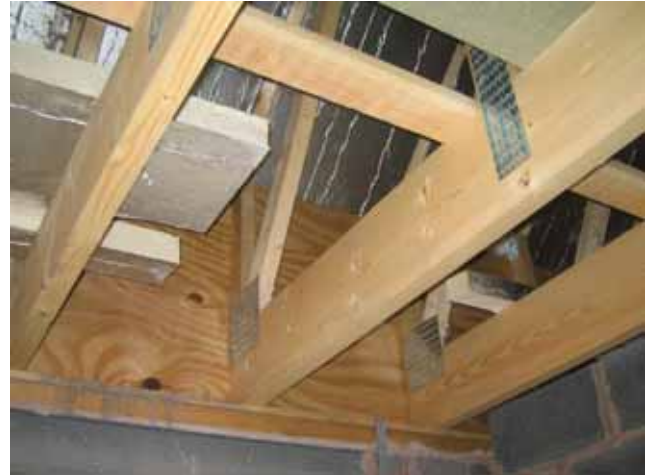
Figure 88 - Attic Truss Viewed from Below
