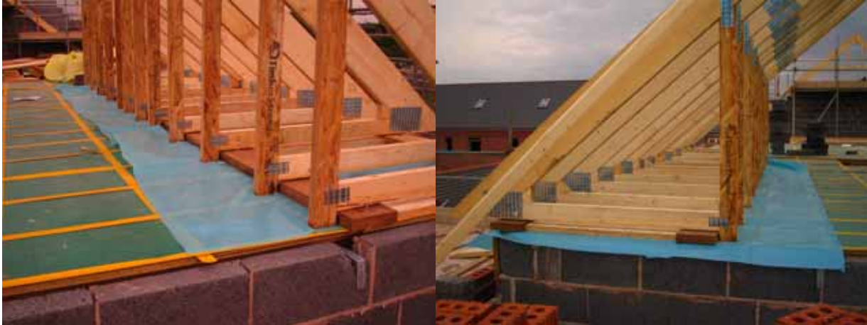
Figure 85 - Polythene Sheet Air Barrier under Roof Truss in Redrow Room-in-Roof Property
