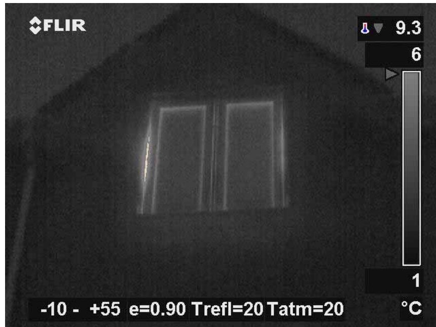
Figure 104 - Thermal Image Showing Heat Loss through Window Trickle Vents
