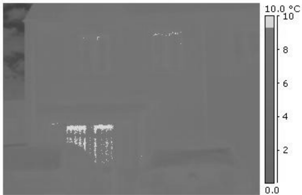
Figure 103 - External Thermal Image of Plot 13 Showing Study in Top Right Corner
