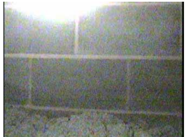
Figure 18 Photo Bottom Attic Wall 401-402
