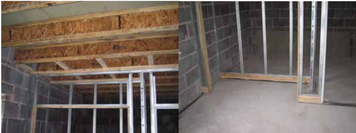
Figure 82 - Timber Studs at Top and Bottom of Steel Frame Partitioning
