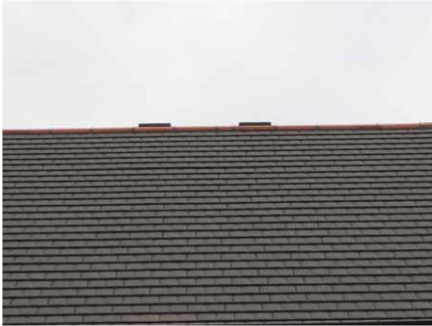
Figure 7 – Ridge Vent on Bryant Property
