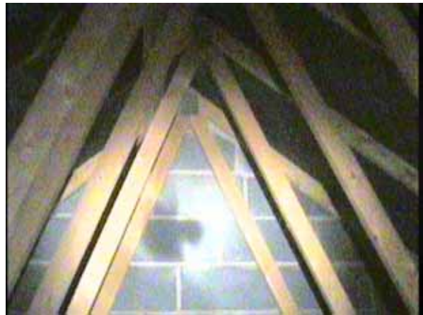
Figure 26 Photo Top Attic Wall 403-402
