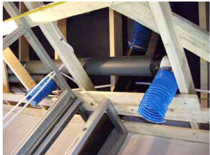
Figure 81 - Partitioning Erected before Ceiling
