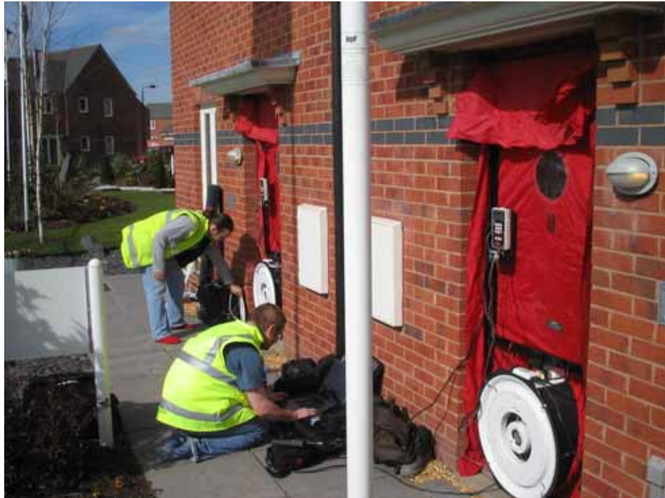
Figure 46 - Photograph of Inter-dwelling Pressure Test using Two Blower Doors
