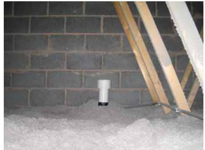
Figure 16 Photograph Plot 13 Attic Gable Wall
