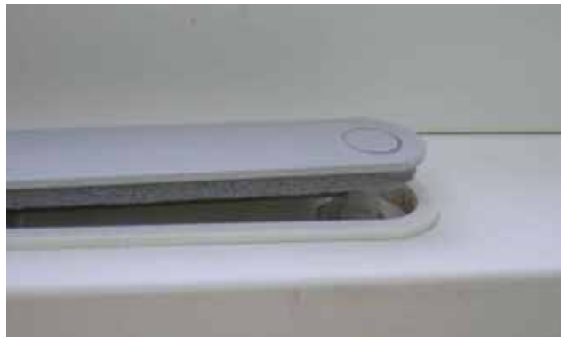
Figure 47 - Trickle Vent on Rationel Window showing Foam Seal
