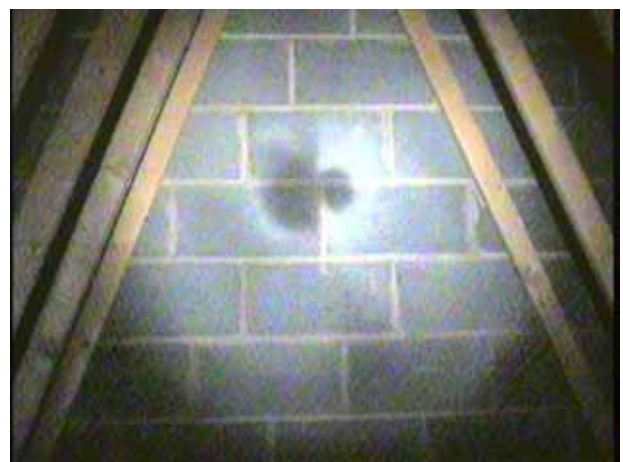
Figure 24 Photo Middle Attic Wall 403-402
