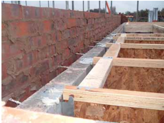
Figure 94 - Intermediate Floor Being Installed on Joist Hangers
