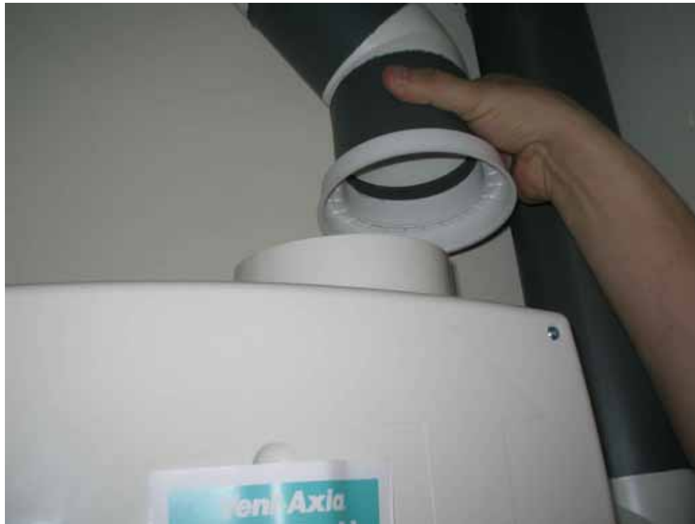
Figure 4 – Disconnecting Outlet Duct
