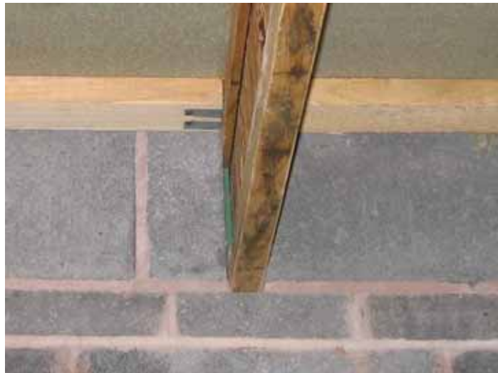
Figure 96 - Built in I-Beam with Foam Insert
