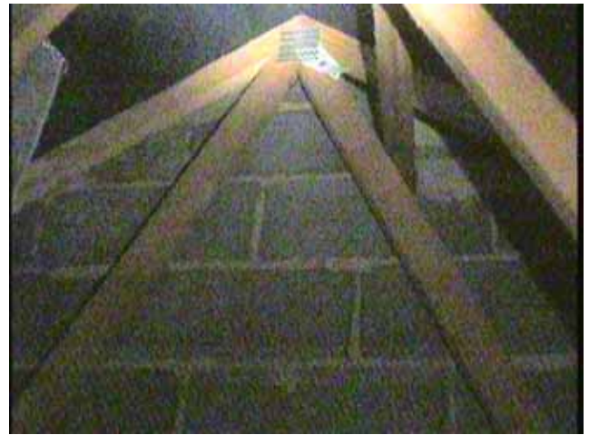
Figure 20 Photo Top Attic Wall 401-402
