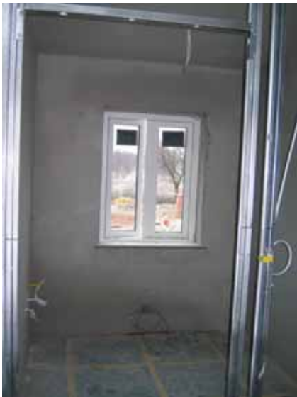
Figure 80 - Plot 13 Ceiling Erected before Partitions
