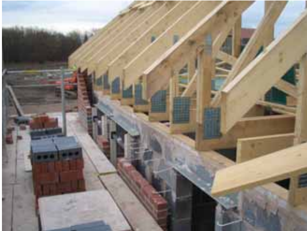
Figure 87 - Attic Truss at Stamford Brook
