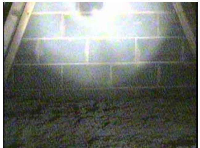
Figure 22 Photo Bottom Attic Wall 403-402
