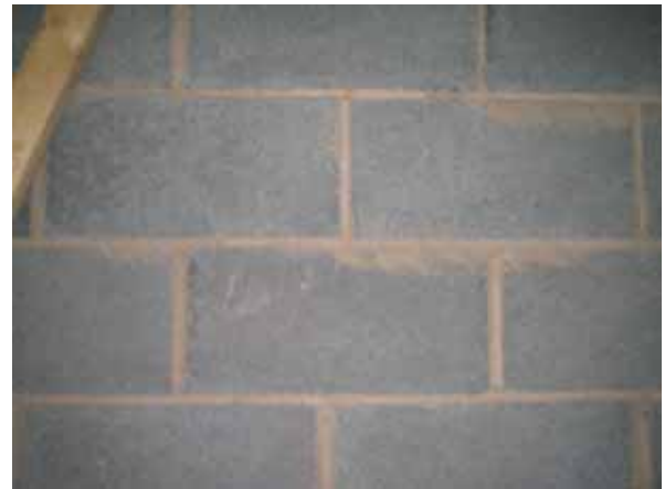
Figure 14 Photograph of Plot 13 Attic Party Wall
