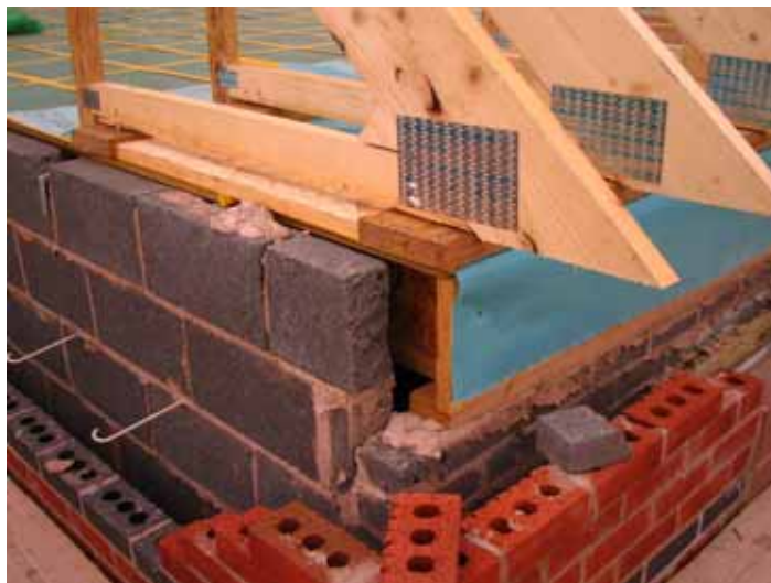
Figure 86 - Polythene Sheet Air Barrier in Room-in-Roof Dwelling
