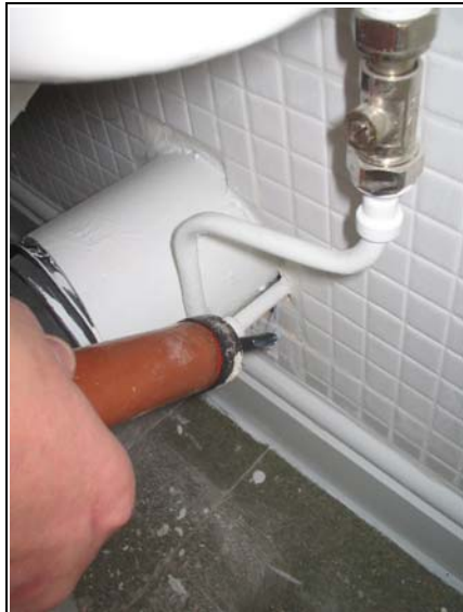
Figure 30. Detected air leakage at plumbing penetrations.
