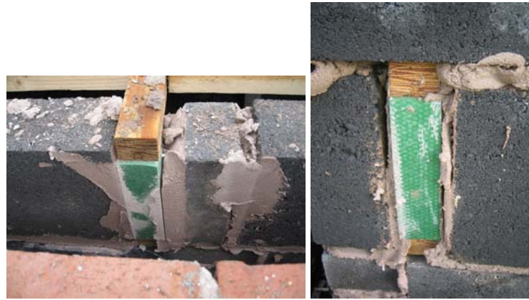
Figure 56. Foam end caps fitted to joists.
