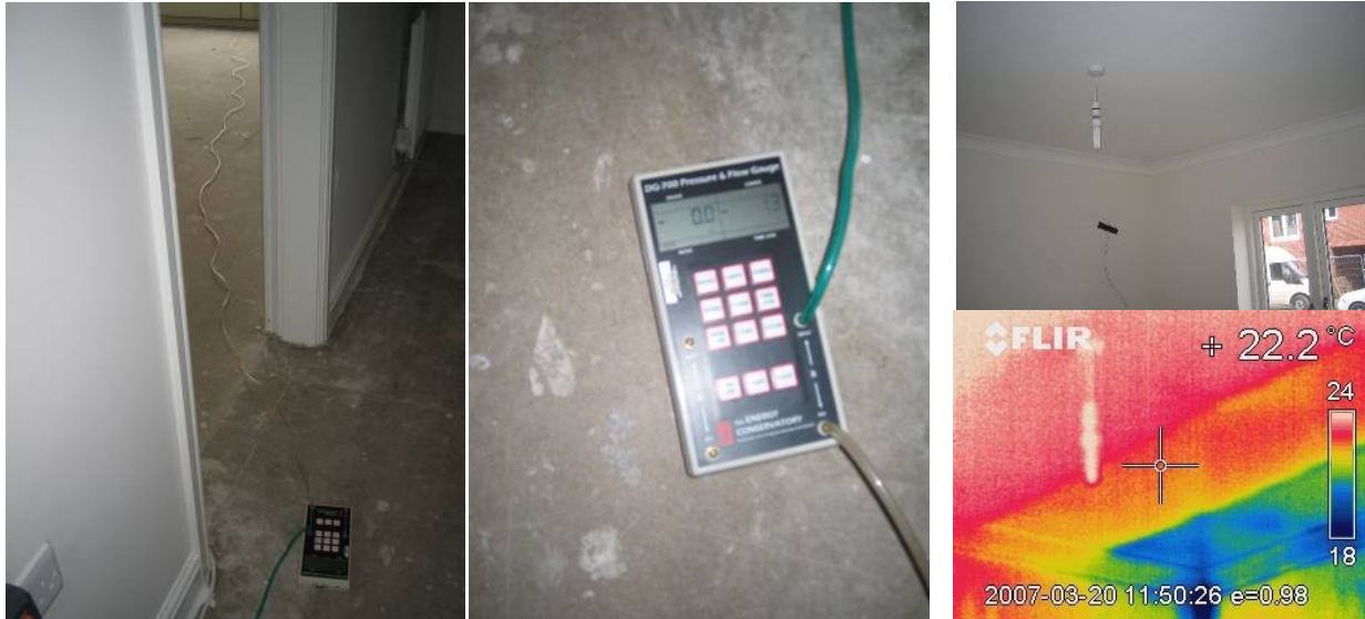
Measurement of pressure differential across the dwelling
