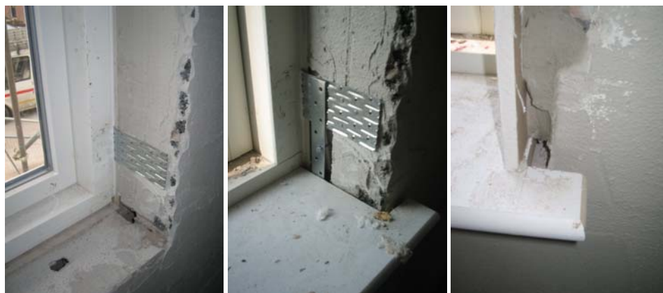
Figure 60. Window sills at various stages of construction.
