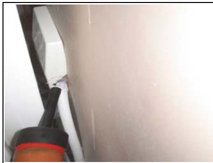
Figure 31. Air leakage detected around radiator pipework.
