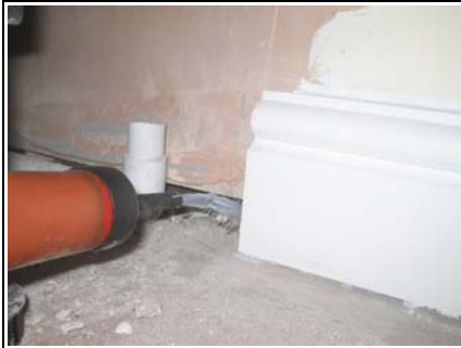
Figure 24. Air leakage at the ground floor/wall junctions.
