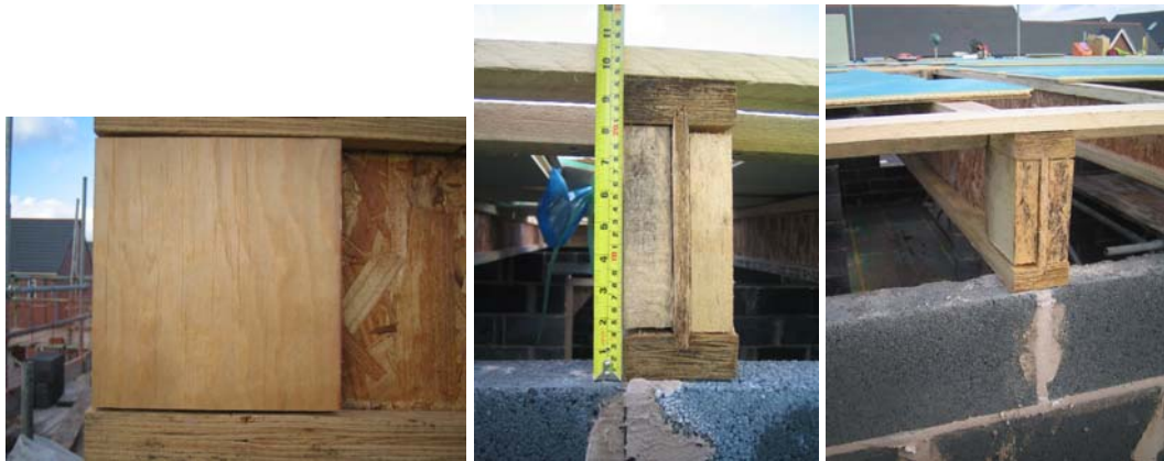
Figure 55. Web stiffeners in plots B119, B120 and B121.
