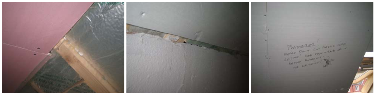
Membrane not linked to ceiling boarding
