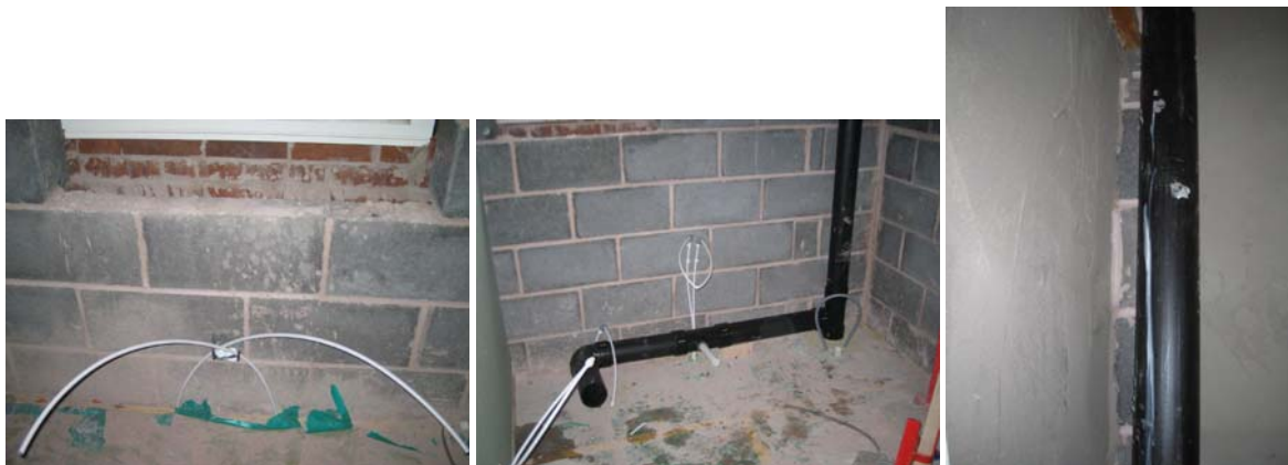
Figure 47. 1 st fix plumbing installations in plots B117 and R110.
