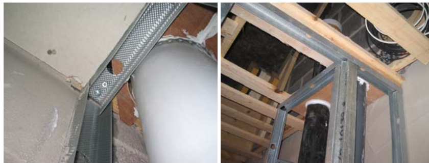
Plywood plate at intermediate floor
