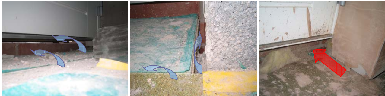
Figure 65. Potential thermal bridge and air leakage paths in plots R110 and R111
