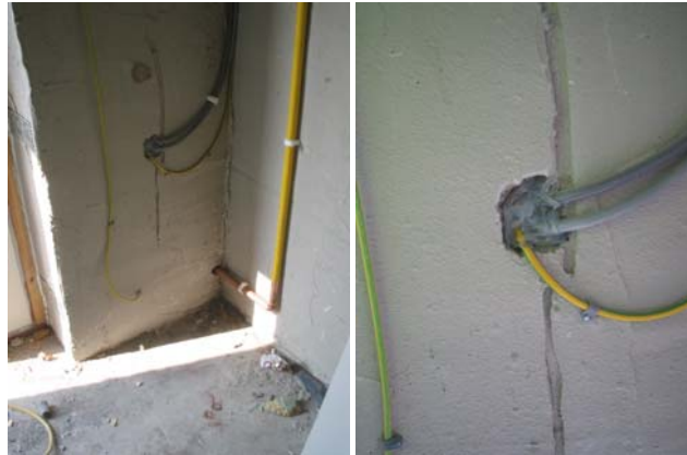
Figure 94. Sealing of the cables to the meter box in plot B120.
