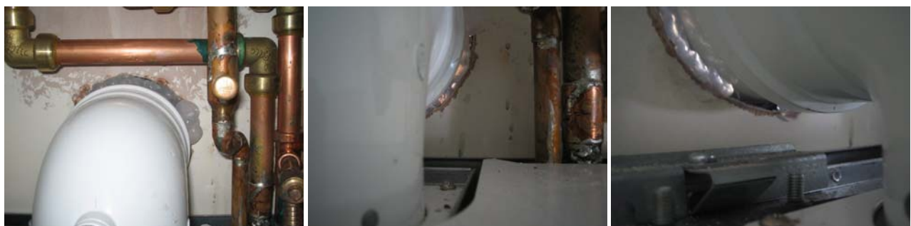
Figure 96. Internal sealing of the boiler flue in plot B121.
