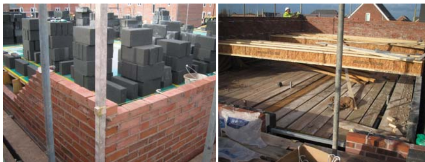
Figure 53. Intermediate floor construction – external leaf built before inner leaf.
