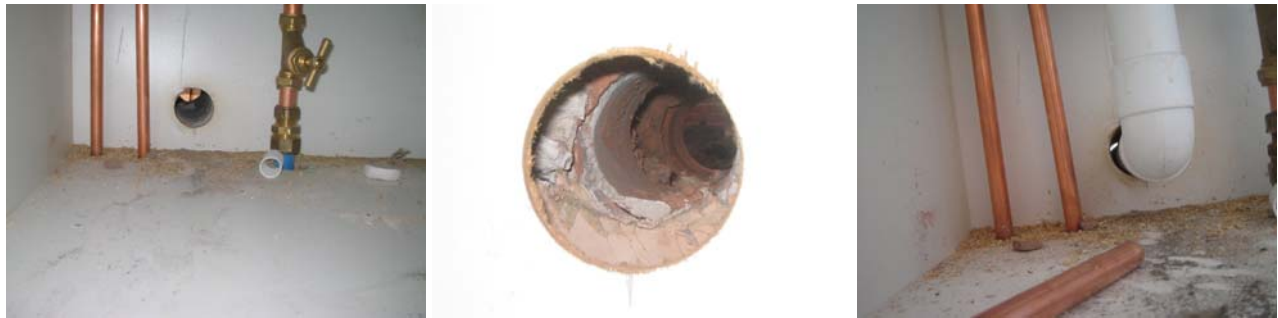
Figure 97. Kitchen sink waste pipe installation in plot R111.
