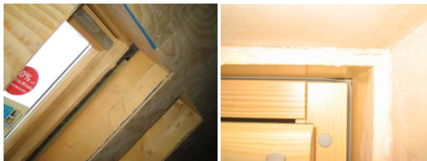
Figure 93. Rooflights in plots R116 and B119.
