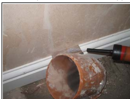
Figure 23. Air leakage around ground floor service penetrations.
