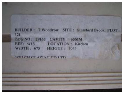
Window former for the correct plot but wrong room
