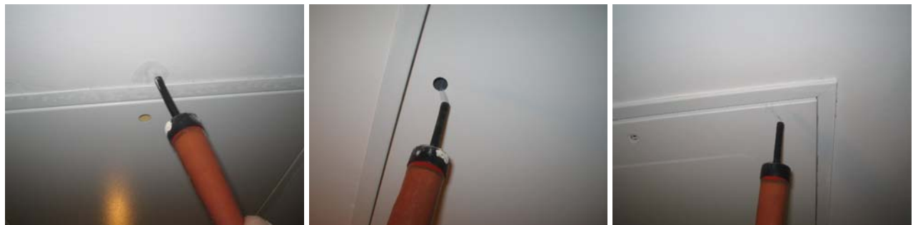
Around the loft hatch surround in plot B120
