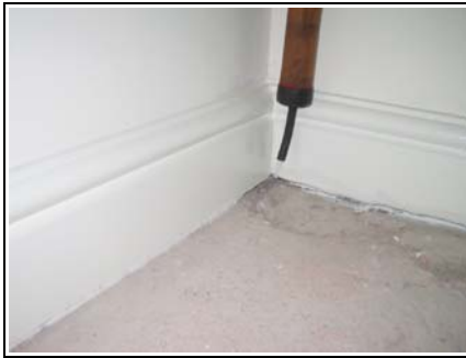
Figure 24. Air leakage at the ground floor/wall junctions.
