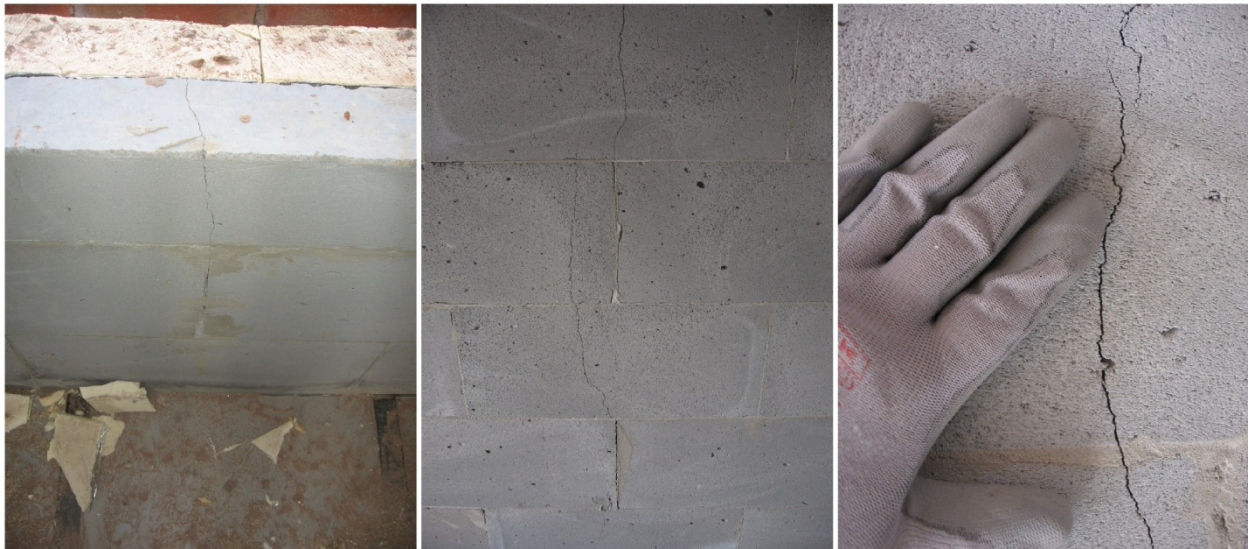
Figure 5 Cracking of the blocks in the masonry prototype.
