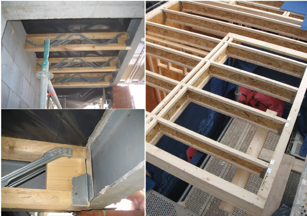
Figure 2 Front canopies in the A1 and A2 prototypes during construction.
