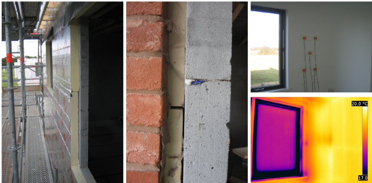
Figure 17 The masonry prototype 1 st floor rear wall (North façade), showing gaps in the insulation, heat flux sensor placement, and thermal image captured during coheating.
