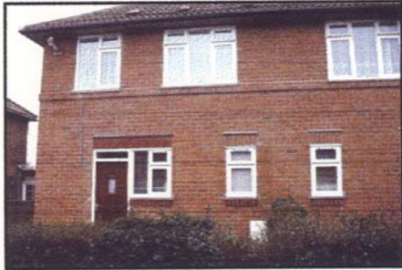
Bell Farm A from front. Photograph for reference.
