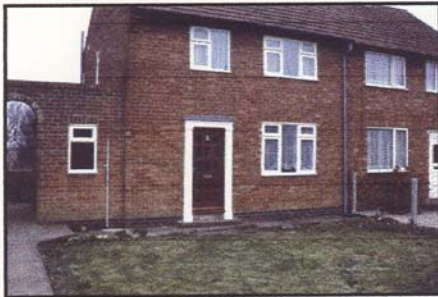
Chapelfield A from front. Photograph for reference.
