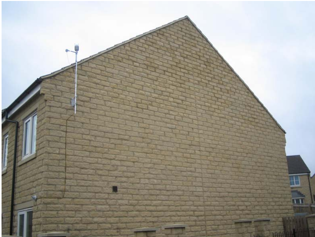
Figure 2 Coheating test weather station installed on gable wall.
