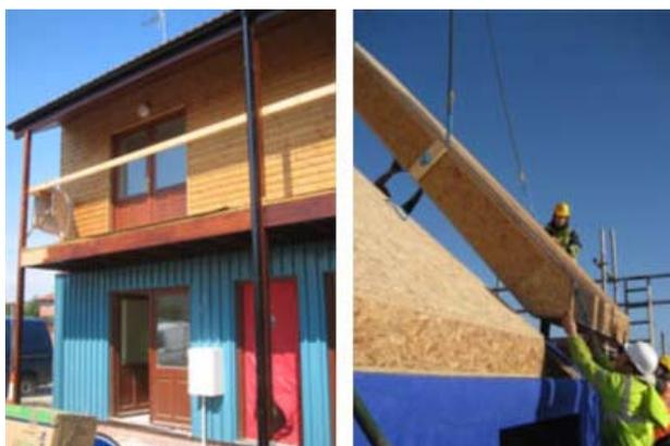
External walls clad in timber and the composite timber-frame roof panels being craned into position [Source: Constructive Individuals, 2008]
