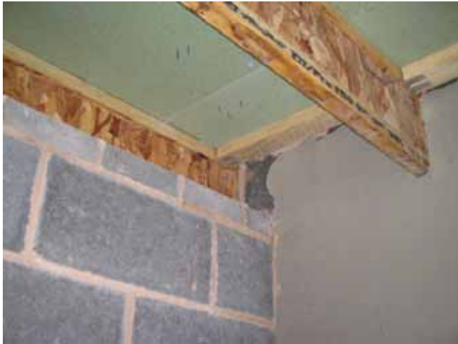
Figure 10: Parging around I-beams.
