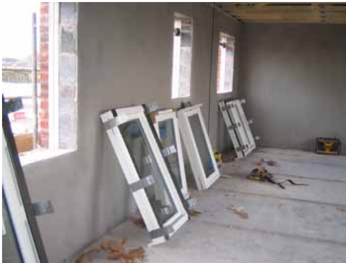
Figure 6: Timber, high-performance, double-glazed windows.
