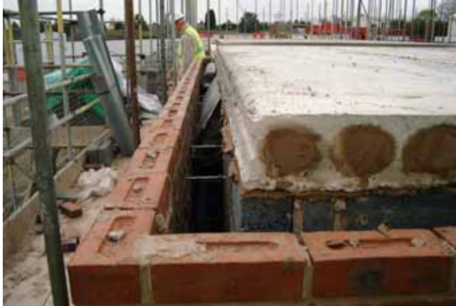
Figure 5: Concrete floor slabs.
