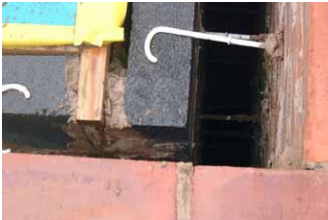
Figure 4: Masonry wall construction showing plastic wall ties.
