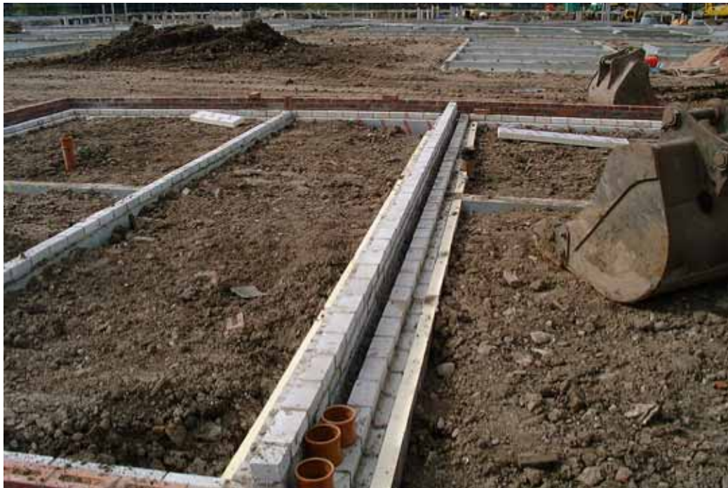
Figure 5: Unnecessary insulation.
