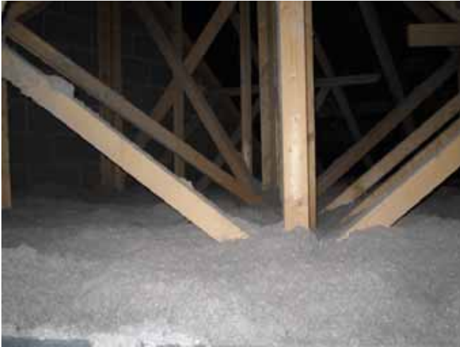
Figure 14: Cellulose roof insulation fitted closely around truss members.
