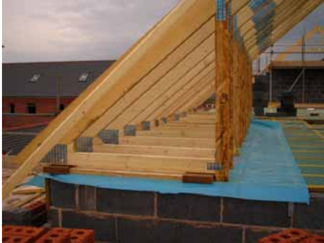
Figure 8: Room-in-the-roof attic trusses showing DPM (blue) air barrier.
