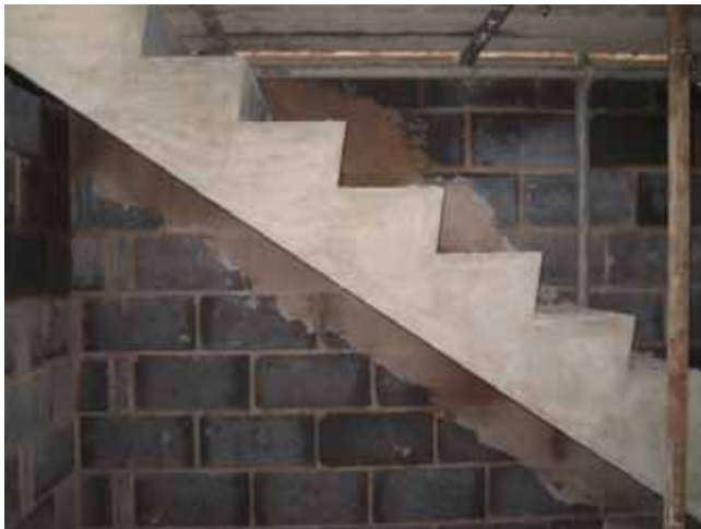
Figure 11: Parging wall before fitting stairs.
