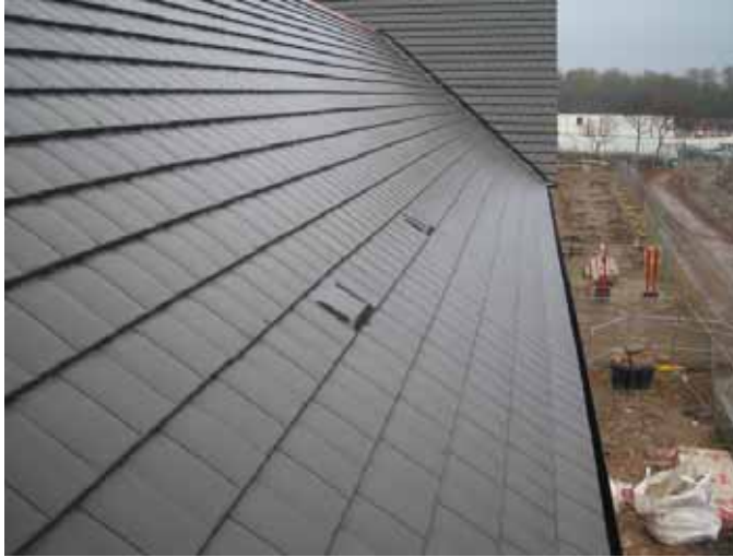
Figure 15: Roof tile terminals for the ventilation ducting.
