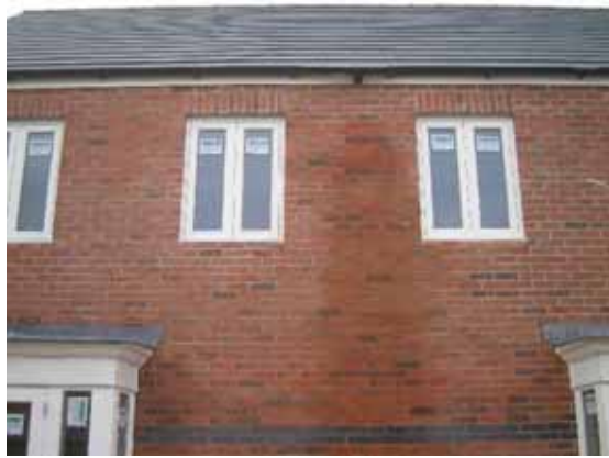
Figure 39 – Rear Wall of Bryant Plot 116-117 – Horizontal Sock Removed
