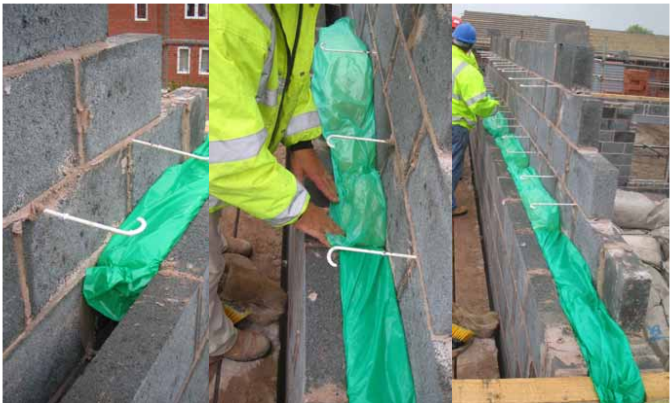
Figure 9 - Installation of Cavity Socks
