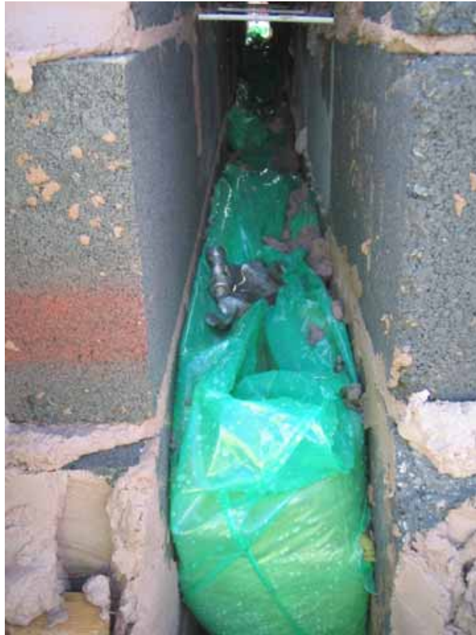
Figure 1 - Trial Installation of Horizontal Cavity Sock in Party Wall
