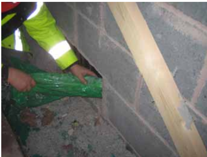
Figure 15 - Removing Cavity Sock
