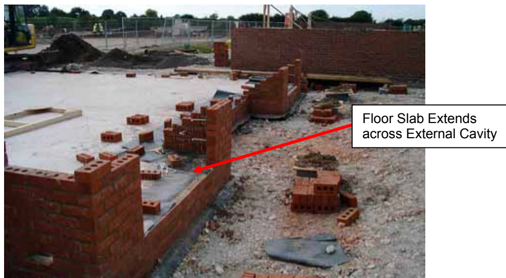
Figure 82 – Ground Floor of Bryant Plots 13 and 14 under Construction
