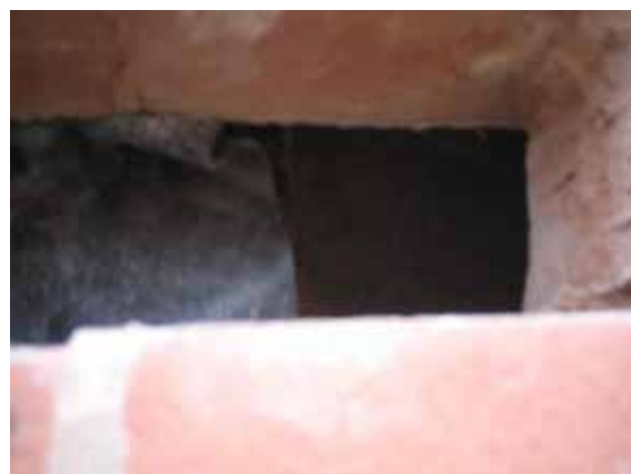
Figure 40 – Missing Insulation in Cavity of Rear Wall of Bryant Plots 116-117
