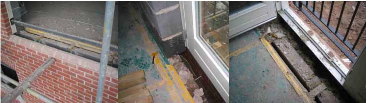
Figure 67 – Construction of Juliet Balcony Threshold Detail
