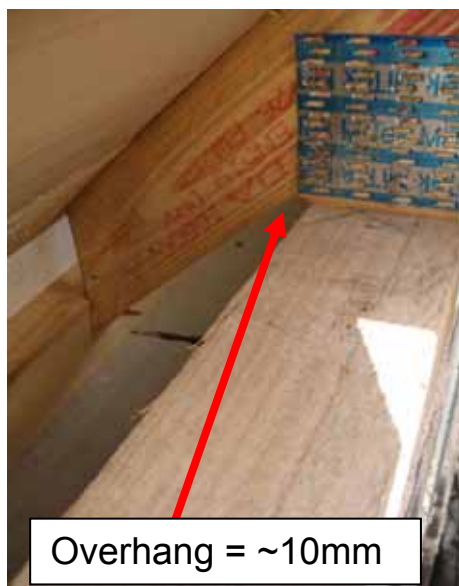
Figure 65 – Roof Truss Overhang at Wall Plate
