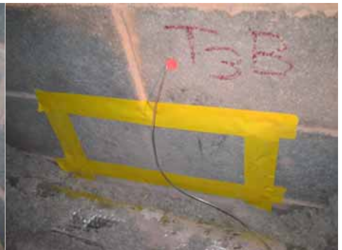
Figure 16 - Block Replaced and Joints Taped Over
