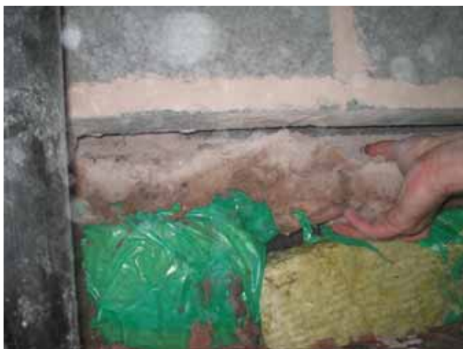
Figure 48 – Mortar Layer on Top of Sock – Redrow Figure 49 – Mortar Covered Sock - Redrow
