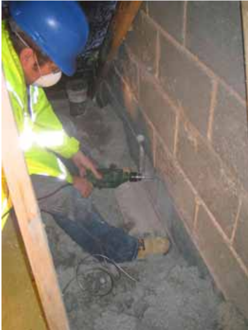
Figure 13 - Drilling out Mortar around Block
