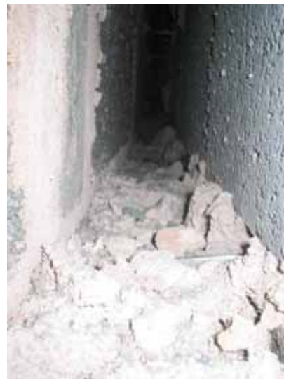
Figure 48 – Mortar Layer on Top of Sock – Redrow Figure 49 – Mortar Covered Sock - Redrow
