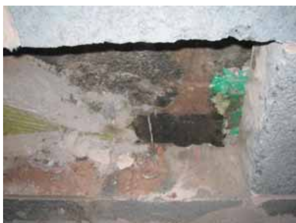
Figure 50 – Damaged Sock – Redrow Figure 51 – Gap between Vertical & Horizontal Sock
