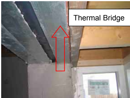
Figure 69 – Bay Window Head before Boarding
