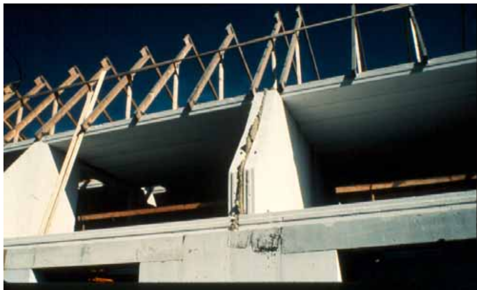
Figure 78 – Fully Filled Party Wall Cavity in Sweden (© R. Lowe and D. Olivier 1980)
