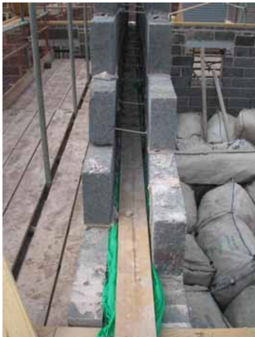
Figure 11 - Sock Protected from Mortar Spots
