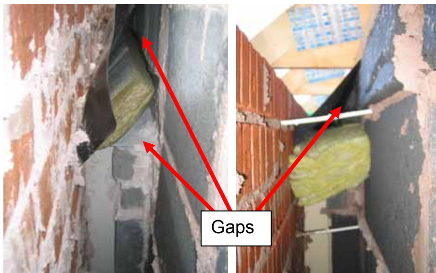
Figure 60 – Insulation underneath Cavity Trays at Window Heads
