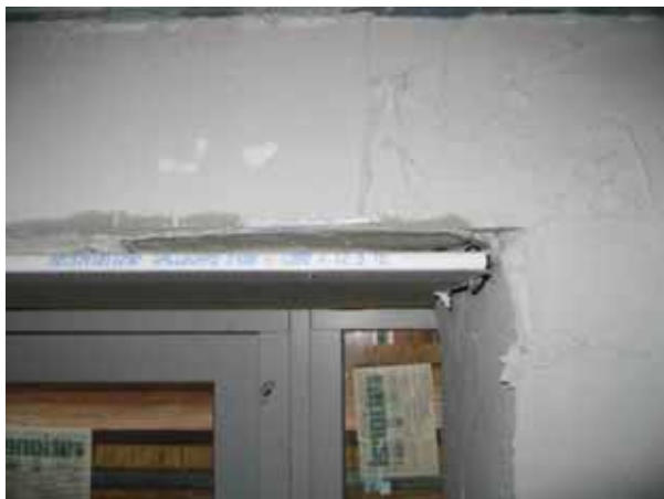
Figure 73 – Uninsulated Reveal Board in Bay Window
