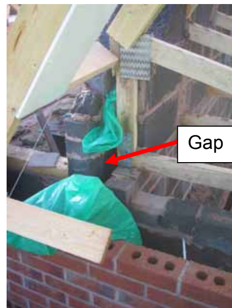
Figure 57 – Gap between Vertical and Horizontal Socks
