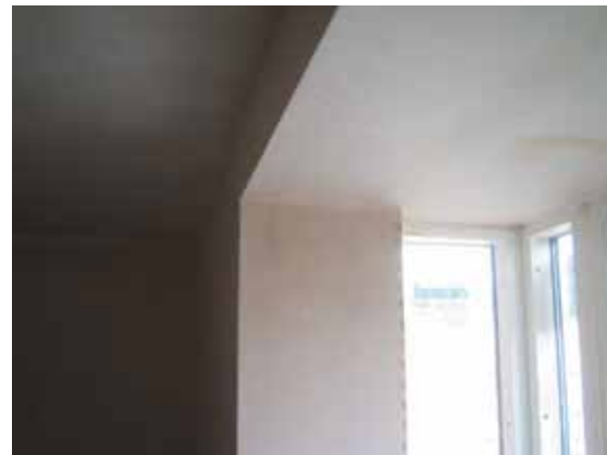
Figure 70 – Completed Bay Window
