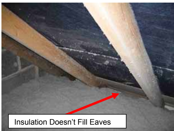
Figure 74 – Loft Insulation at Eaves
