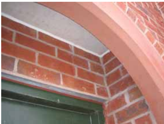
Figure 45 – Thermal Bridge at Front Door Recess – Redrow 110.
