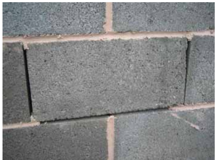
Figure 12 - Removable Block in Party Wall
