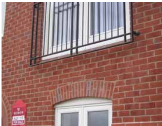
Figure 44 – Thermal Bridge at Juliet Balcony Threshold – Redrow Plots 110
