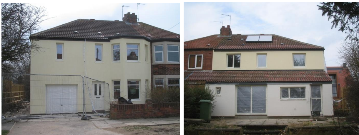
Figure 3 Front and rear elevations following stage 2 renovations
