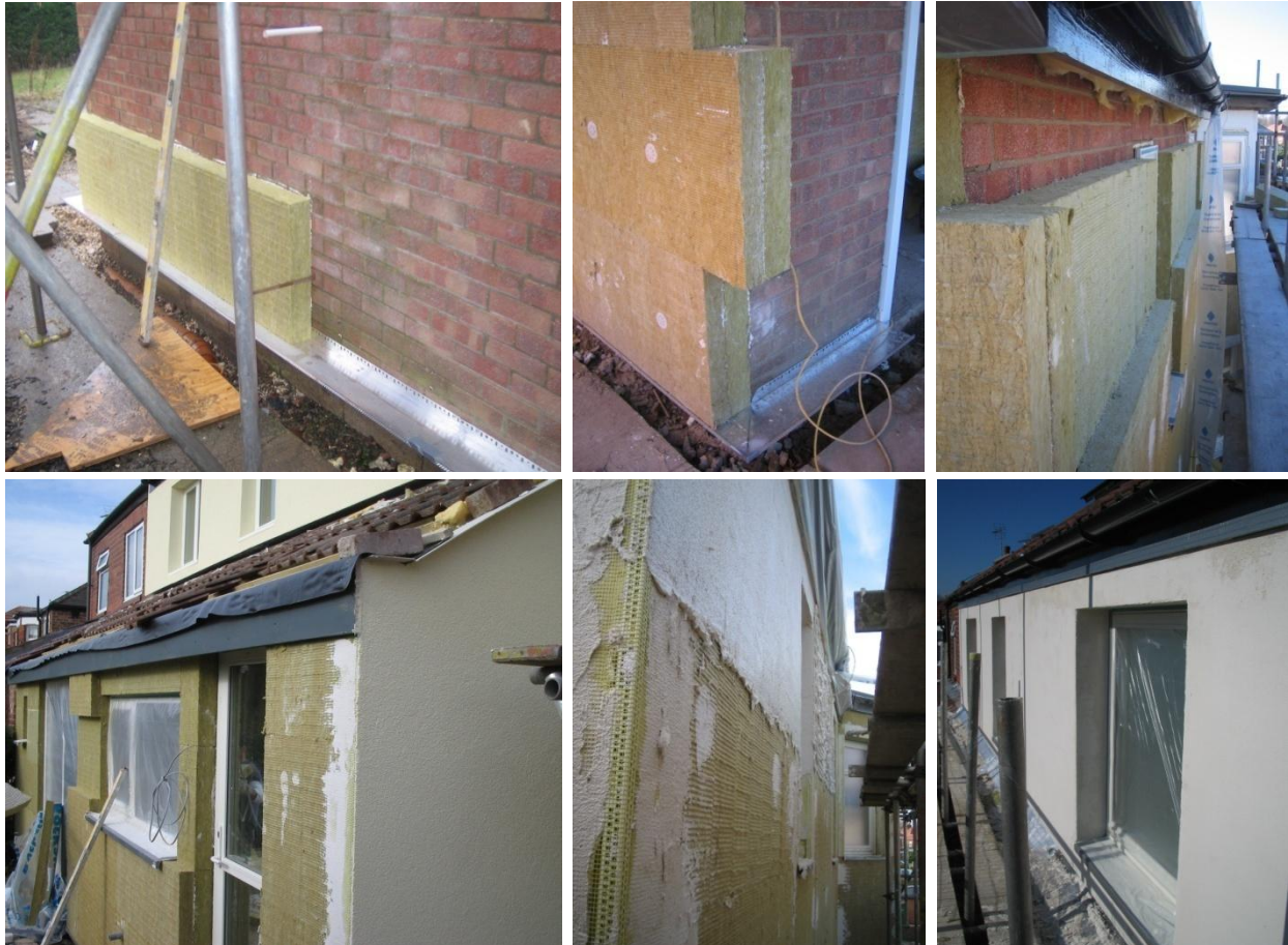
Figure 22 EWI installation, February to March 2010.
