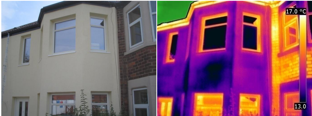
Figure 27 Finished party wall EWI detail and thermal image, front elevation.
