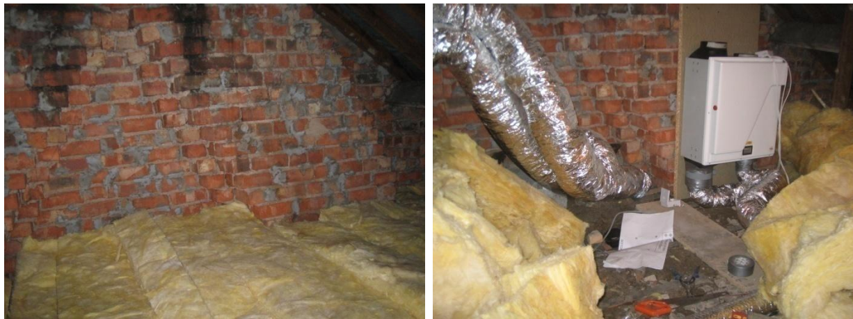
Figure 34 Loft insulation when laid (07-Dec-09) and after MVHR unit installation (02-Mar-10).
