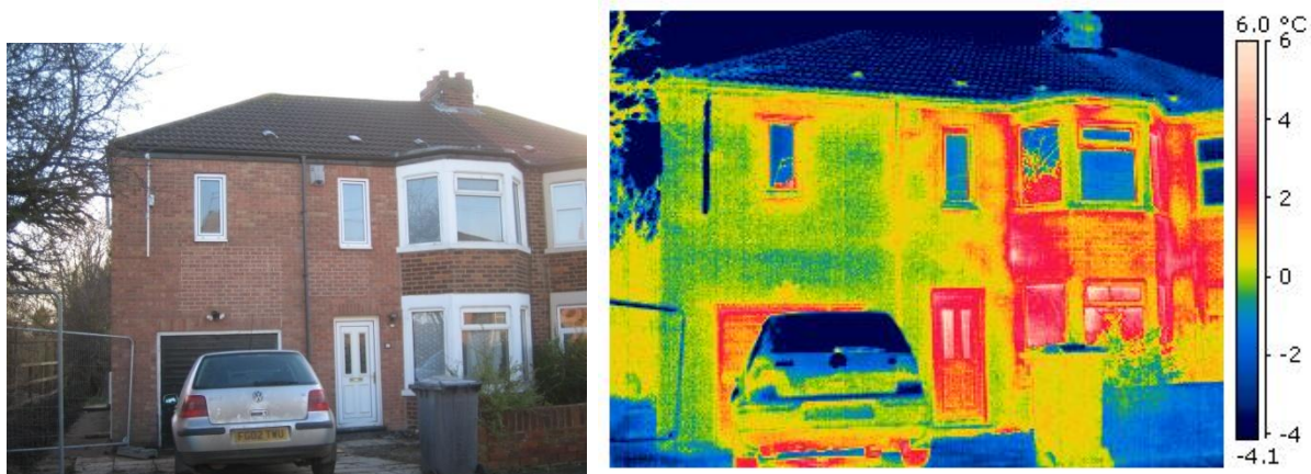
Figure 5 Front elevation during coheating test 2, 17-Dec-09, following cavity wall insulation installation.
