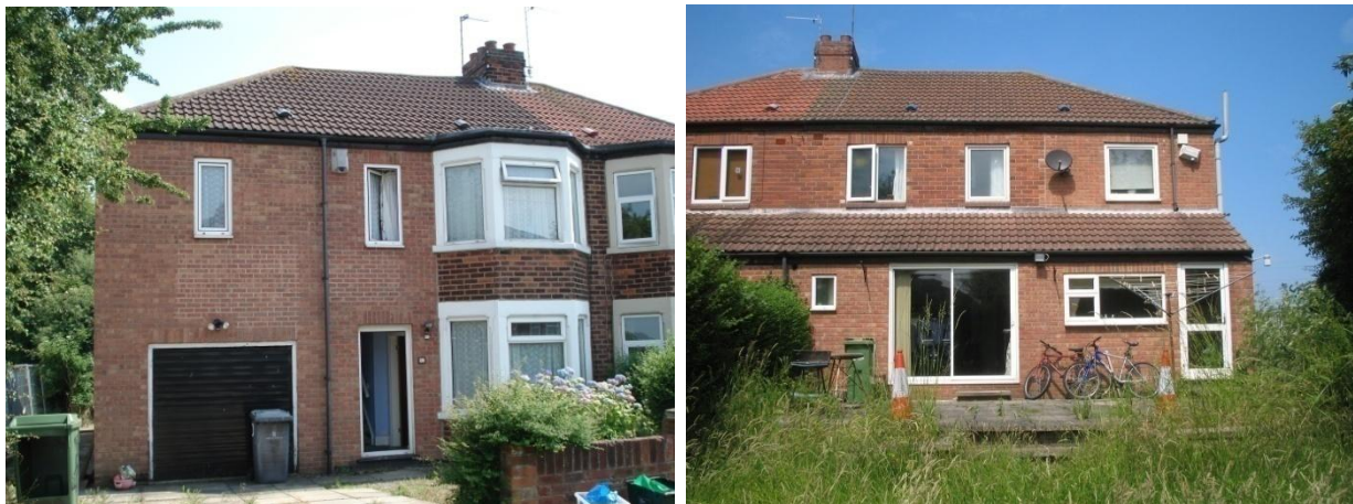
Figure 2 Front and rear elevations prior to any renovation work.
