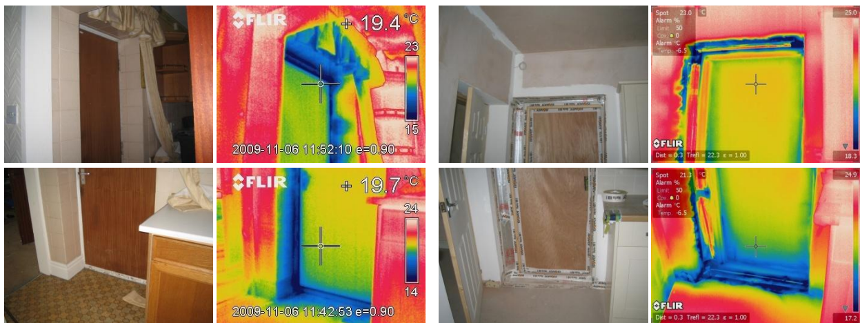
Figure 40 Infiltration around the door between the kitchen and the garage at the November 2009 and March 2010 pressurisation tests.
