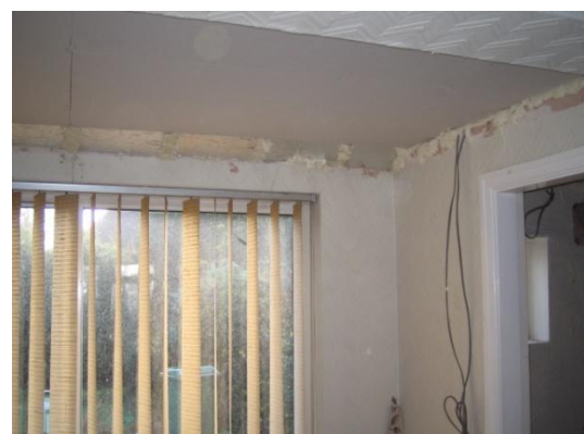
Figure 14 Eaves at the rear extension during the 2 nd coheating test with the insulation and air barrier relocated to rafter level.
