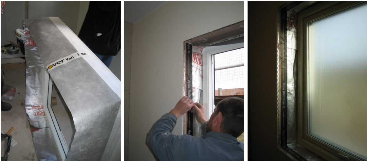
Figure 31 Installation of triple glazed replacement windows showing the air barrier.
