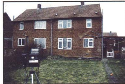
Chapelfield A from back. Note boiler flue to left of kitchen window, and infra-red camera in foreground.
