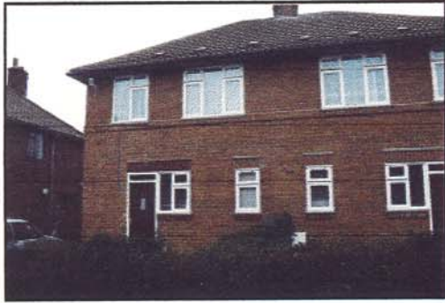
Bell Farm A&B from front. Note external temperature sensor at top left hand corner.
