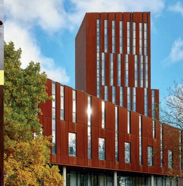
Broadcasting Place, exterior
