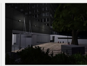
H Building 2016, October
