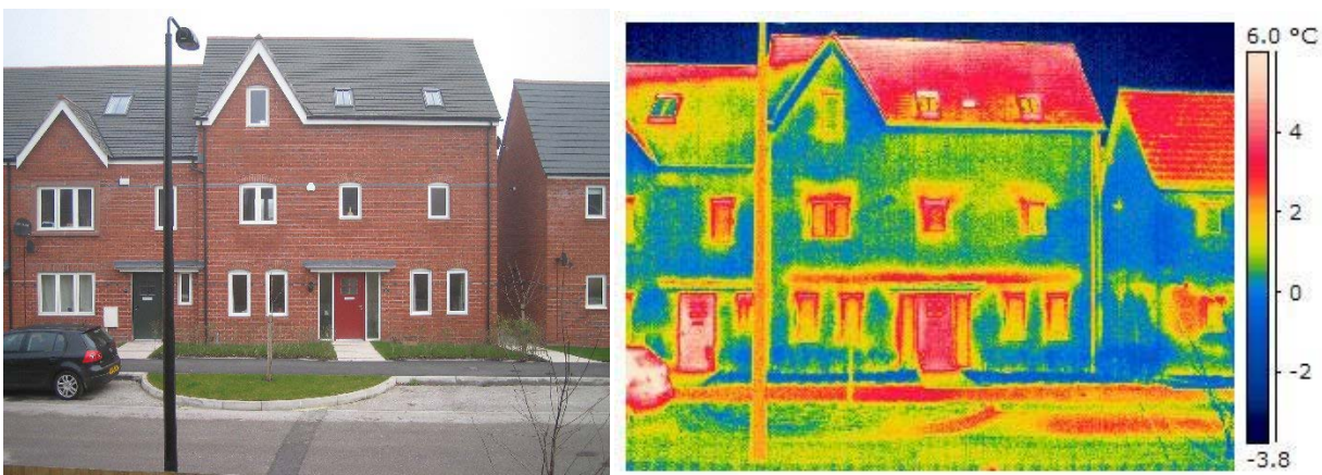
Whole building thermography from Stamford Brook study (Leeds Metropolitan University, UK)
